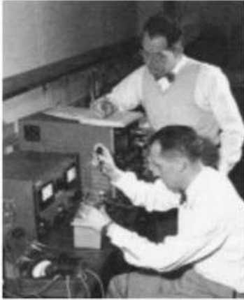
Dr. Ian Munro Ross (front) and G. C. Dacey jointly developed an experimental procedure for measuring the characteristics of a field-effect transistor in 1955. (Courtesy of AT&T Archives.)
